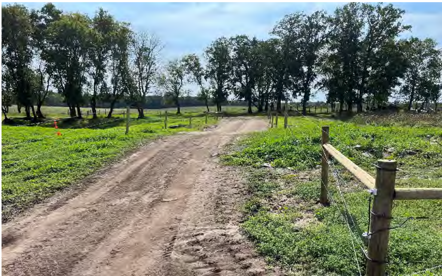
View looking southward at completed livestock crossing
