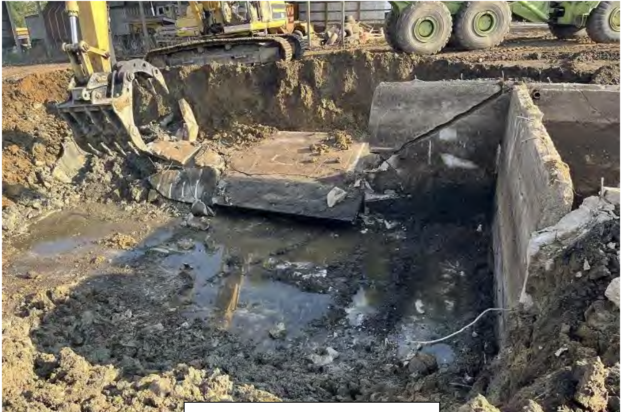
Removal of Concrete Pit
