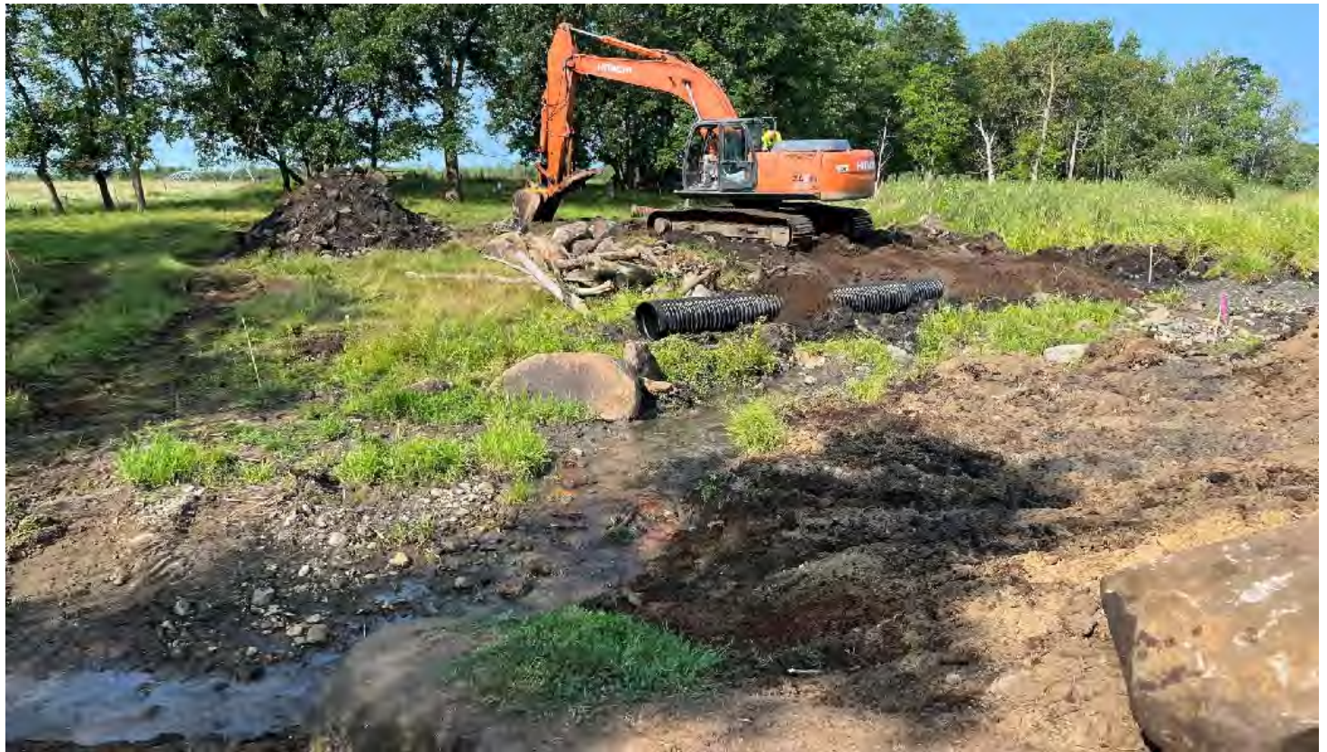
Contractor Installing culvert
