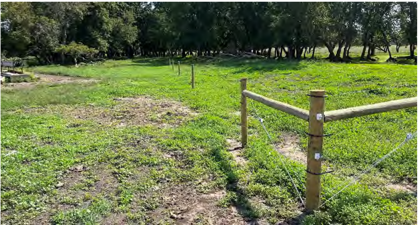
High tensile electric fence was installed along stream west and east of crossing on property
