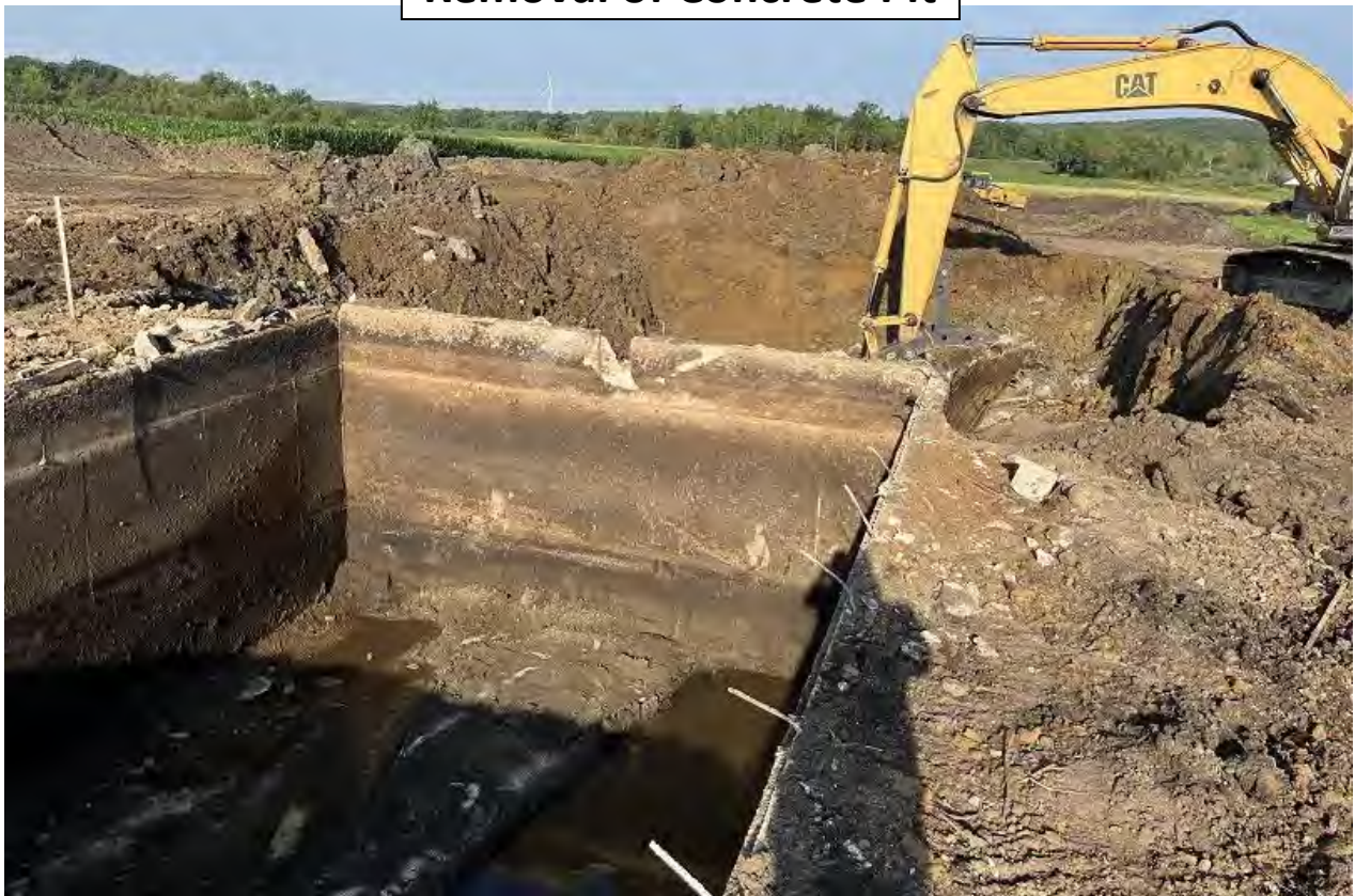
Removal of Concrete Pit
